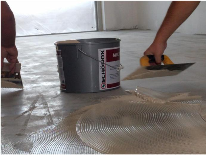
**Schönox® Multi Object** offers excellent coverage (features low consumption), is suitable for internal use (does not contain solvents, carries VOC certifications), is a certified surface-cleaning product (easy to maintain) and is suitable for application in combination with underfloor heating systems and stress from office chair wheels. The total surface for self leveling mortars & LVT tiles was 10.000m<sup>2</sup>.
