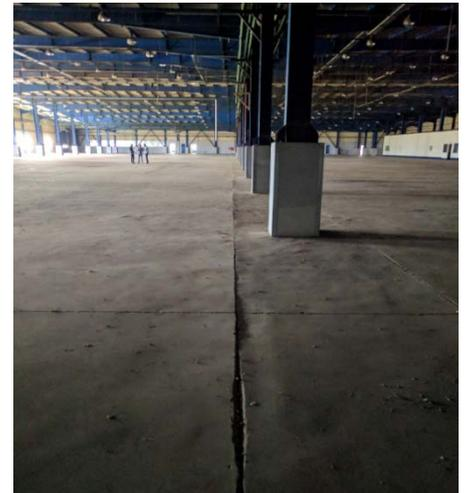
Consequently, the existing flooring system was stripped and the surface was prepared using shot blasting in conjunction with abrasive rotary equipment.
