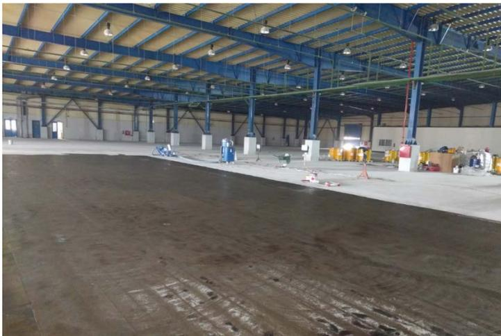
Subsequently, the **Sikafloor® MultiDur ES-20** system was implemented. **Sikafloor® MultiDur ES-20** is a color, self-leveling epoxy-based flooring system that forms wear-resistant, smooth, glossy finish with limited maintenance requirements. It is suitable for moderate to heavy stress conditions. **Sikafloor® MultiDur ES-20** forms a smooth gloss finish and is applied at nominal thickness of 1,5–3,0 mm.
