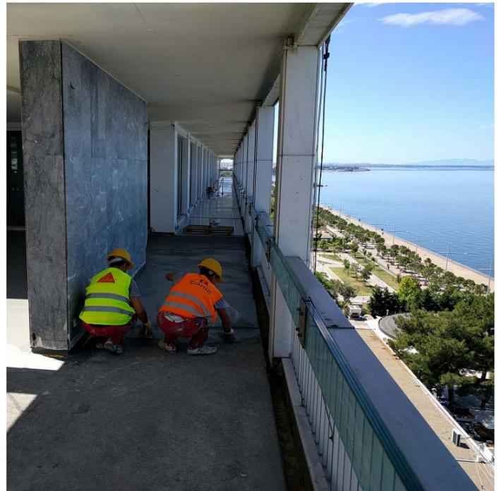
product prior to tile bonding using C2 (acc. to EN 12004) cementitious tile adhesives. At the joints and edges of the surface, the special waterproofing tape **Sika® SealTape-S** was encapsulated between layers of **Sikalastic®-1k** to ensure full watertightness.
