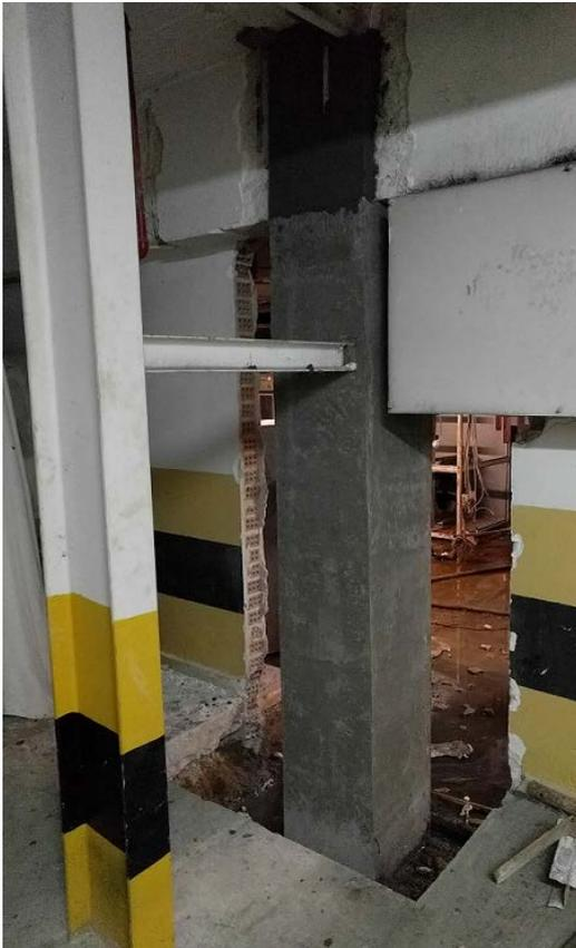
Structural reinforcement was carried out using **SikaWrap®-230 C** woven carbon fiber fabric (unidirectional fibers) bonded using the 2-component **Sikadur®-330** epoxy resin (Dry Application Method). **SikaWrap®-230 C** offers high economic efficiency compared to traditional reinforcement techniques and offers ease of molding as it is adapted to the geometry of the structural member.
