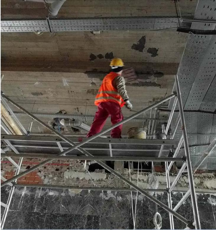
For the restoration of the original section of columns in the basement of the hotel, the 1-component, fibre reinforced, cementitious grout **Sika® MonoTop-634** was used.
