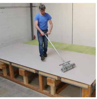
After the membrane is applied, use a water-filled or steel roller to press down the membrane properly to the substrate.
