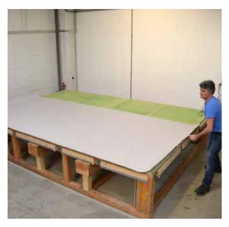
Membrane is rolled out and aligned in the correct position with the correct overlaps.
