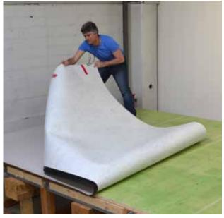
Remove release liner on half of the membrane by drawing off. Adhere the membrane to the substrate. We recommend using a brush or a putty knife to prevent blisters. Execute the same procedure on the other half of the membrane.
