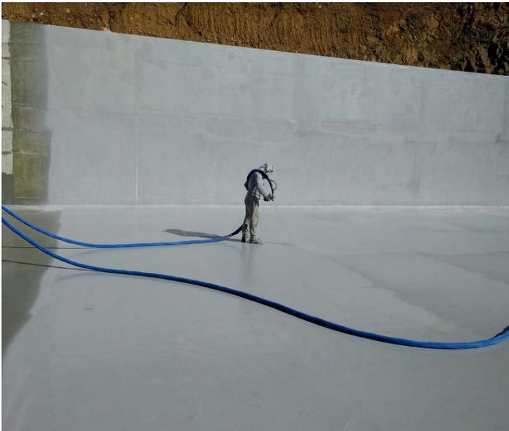
The 2-component acrylic-polyurethane final paint with weather-resistant **SikaCor® EG-5** was applied to the entire surface of the water-free reservoir and exposed to UV radiation (from the height of its upper level water and the handrail, about 1 m below the rim of the tank) in Ral 7035 colour shade.
