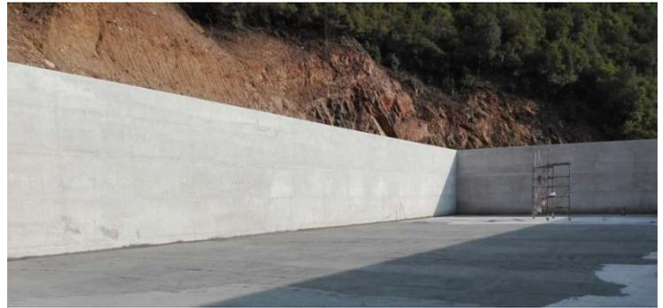
On the perimeter walls, the 2-component **Sikafloor®-161** epoxy primer was applied first, followed by **Sikafloor®-161** scratch coat:
