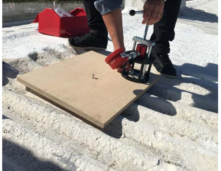
After the quality of the substrate was evaluated, expanded polystyrene insulation boards were applied to flatten the surface and increase the thermal insulation performance of the building. On this substrate the application of the **Sarnafil® TS 77-15** membrane followed, using all the auxiliary products for linear and point support.
