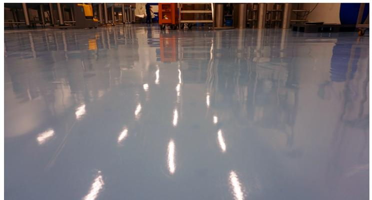
**Sikafloor® MultiDur ES-20** system was also applied to the 1.750m2 surface area where existing epoxy flooring had to be restored. The system was applied to the existing epoxy system, as there was chemical compatibility between the existing and the new system. After the floor was mechanically prepared to ensure proper application of the new system on a stable substrate, **Sikafloor® MultiDur ES-20** was laid.
