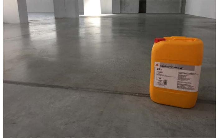
The expansion floor joints were sealed with **Sikaflex®-11 FC<sup>+</sup>**, a 1-component elastic polyurethane sealant.
