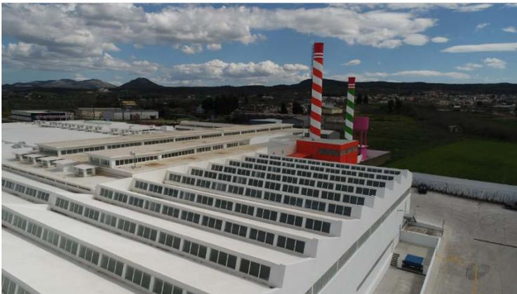
In joints, inverted beams, junctions the **Sikalastic®-612** system was reinforced with **Sika® Reemat Premium** glass fibre mat. **Sikalastic®-621 TC** was applied as a final coating to increase the system's durability and ensure permanent UV reflection. **Sikalastic®-621 TC** is a 1-component, liquid membrane, resistant to ultraviolet radiation (yellowing), while featuring high reflectivity properties (RAL9016).
