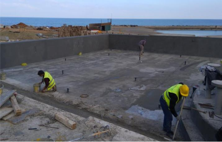
**Sikalastic®-1K** is a 1-component, cementitious, waterproofing mortar, with exceptional crack bridging abilities. It is CE certified and carries Declaration of Performance as concrete protection mortar and as waterproofing mortar for use beneath tiles. **Sikalastic®-1K** was also used for waterproofing beneath tiles for all external verandas and patios.
