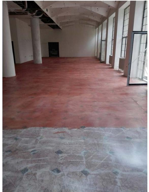
Afterwards, the cementitious levelling mortar **SikaDecor®-803 Nature** was applied, into which the anti-alkali coated glass mesh **Sika® FiberNet** was embedded (in 2 layers).
