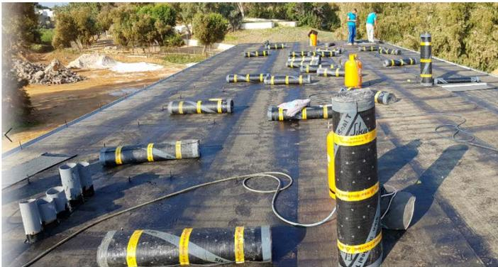
It was then followed by application of **Sika® BituSeal T – 660 MG (-20 °C) HR** bituminous membrane using torch.
