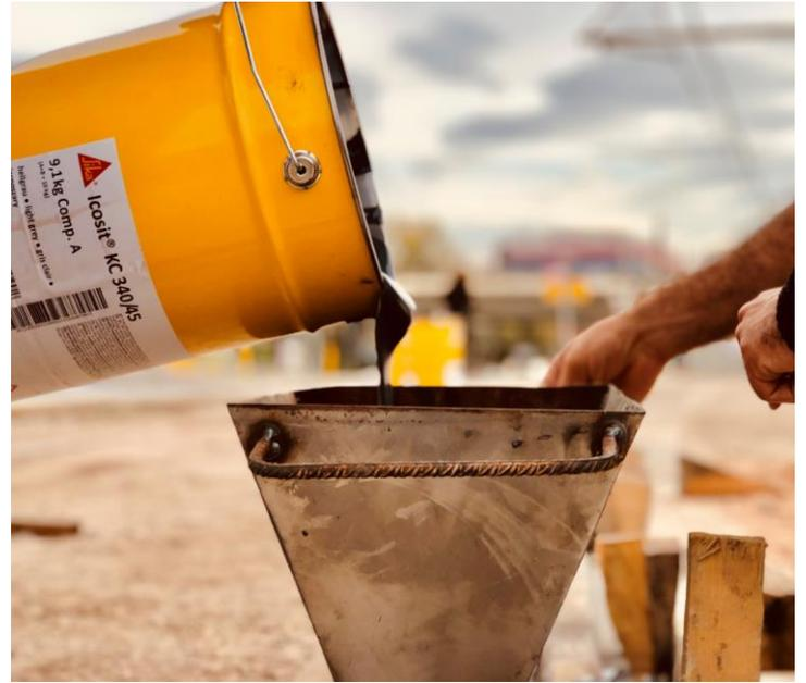
The 2<sup>nd</sup> application phase starts ~12h after the 1<sup>st</sup> phase end and the product is applied on both sides of the rail, in order the full rail embedment up to the required height.
