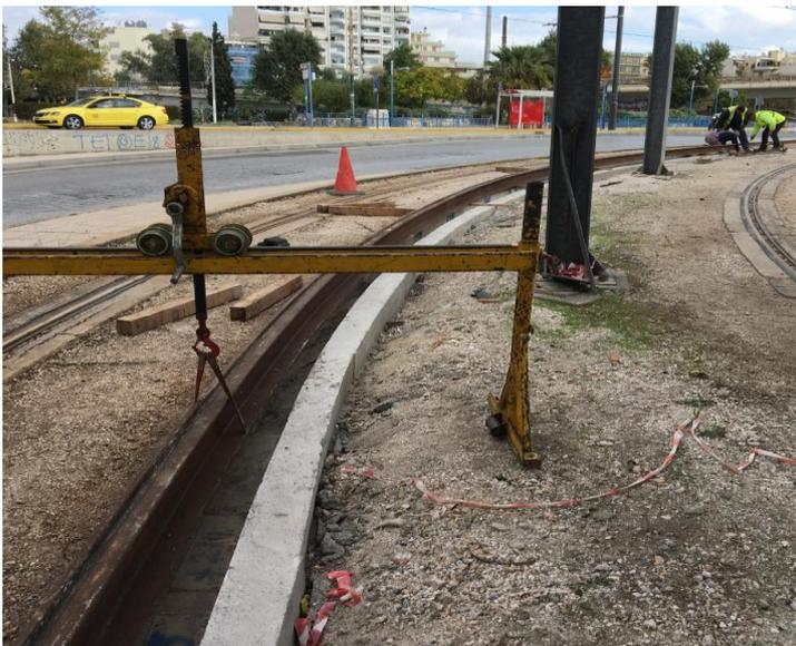
After products' curing, used for the rail box restoration and prior to the installation of the new rail, **Icosit® KC 330 Primer**, 1-component, polyurethane based primer was applied on both concrete and rail.
