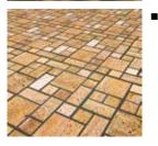
■ **Step 5:** Sika® FastFix-132 PaveFix will start to set in 6 to 12 hours above 15°C in dry conditions. Allow up to 4 days for full set in temperatures between 4°C and 15°C. Contact with rain or moisture can slow the final set.
