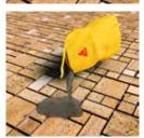
■ Step 3: Use Sika® FastFix-132 PaveFix in small manageable amounts. Avoid spreading over a large area before application. Ensure material is loose by raking through. Do not try to break up and use any small set lumps. Do not add any extra sand.
