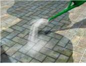
4. Saturate the joints with water using a hose or watering can.
