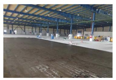
Subsequently, the Sikafloor<sup>®</sup> MultiDur ES-20 system was implemented. Sikafloor<sup>®</sup> MultiDur ES-20 is a color, self-leveling epoxy-based flooring system that forms wear-resistant, smooth, glossy finish with limited maintenance requirements. It is suitable for moderate to heavy stress conditions. Sikafloor<sup>®</sup> MultiDur ES-20 forms a smooth gloss finish and is applied at nominal thickness of 1,5–3,0 mm.
