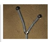
FlexoDrain Substrate drainage system installed to allow the shotcrete application in case of moderate water ingress and protecting the lining from aggressive mountain water.
