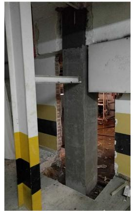
Structural reinforcement was carried out using SikaWrap®-230 C woven carbon fiber fabric (unidirectional fibers) bonded using the 2-component Sikadur®-330 epoxy resin (Dry Application Method). SikaWrap®-230 C offers high economic efficiency compared to traditional reinforcement techniques and offers ease of molding as it is adapted to the geometry of the structural member.
