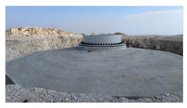
After hardening, on the concrete surfaces the 1-component, anionic asphalt emulsion **Igol®-A** was applied.
