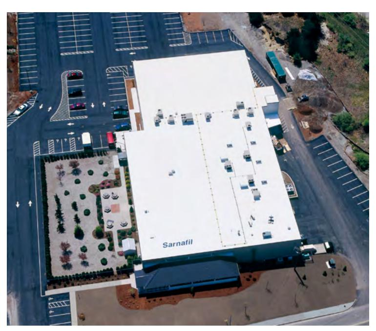
$\mid$  Introduction of EnergySmart white membrane to reduce building energy consumption due to its high reflectivity of sunlight
