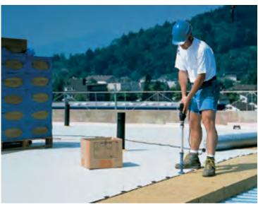
1979 | Mechanically fastened roofing system is introduced
