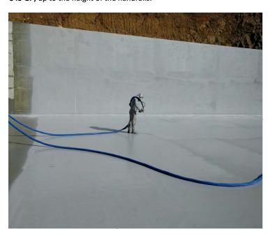
The 2-component acrylic-polyurethane final paint with weather-resistant **SikaCor® EG-5** was applied to the entire surface of the water-free reservoir and exposed to UV ratiation (from the height of its upper level water and the handrail, about 1 m below the rim of the tank) in Ral 7035 colour shade.
