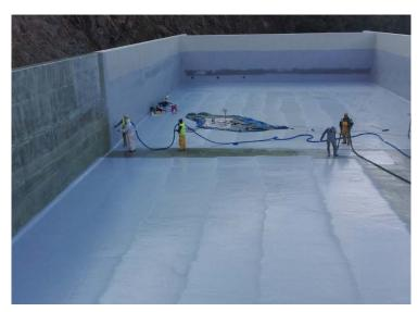
Then water jetting followed for dust removal and application of the 3-component micromortar based on cement and epoxy resins **Sikagard®-720 EpoCem®** for surface smoothing of the floor of the reservoir:
