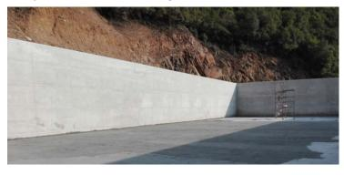
On the perimeter walls, the 2-component **Sikafloor®-161** epoxy primer was applied first, followed by **Sikafloor®-161** scratch coat:
