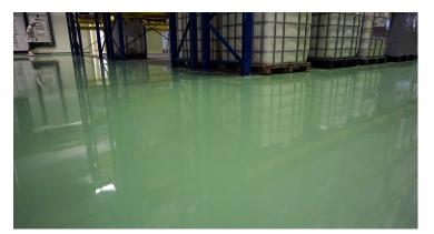
For an intermediate area, where frequent washing takes place, the smooth, glossy, hybrid (cement/polyurethane) flooring system Sikafloor® PurCem® HS-21 Gloss was applied. Sikafloor® PurCem® HS-21 Gloss system features good chemical resistance, dense structure, scratch-resistant surface, high mechanical strength, low dirt pick-up and is easy to clean and maintain. The system features a multitude of certificates, in terms of ease of cleaning & minimal volatile emissions.
