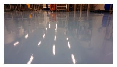
Sikafloor® MultiDur ES-20 system was also applied to the 1.750m2 surface area where existing epoxy flooring had to be restored. The system was applied to the existing epoxy system, as there was chemical compatibility between the existing and the new system. After the floor was mechanically prepared to ensure proper application of the new system on a stable substrate, Sikafloor® MultiDur ES-20 was laid.
