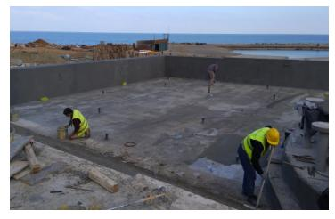
**Sikalastic®-1K** is a 1-component, cementitious, waterproofing mortar, with exceptional crack bridging abilities. It is CE certified and carries Declaration of Performance as concrete protection mortar and as waterproofing mortar for use beneath tiles. **Sikalastic®-1K** was also used for waterproofing beneath tiles for all external verandas and patios.
