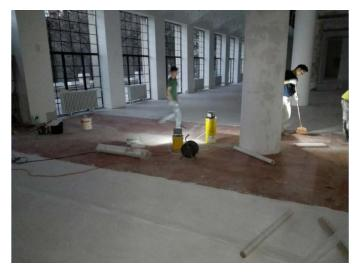
On this reinforced base coat, the fine decorative cementitious micro mortar **SikaDecor®-801 Nature** was applied. The system was completed with the application of the water based, polyurethane, 2-component coating **Sikafloor®-304 W**.
