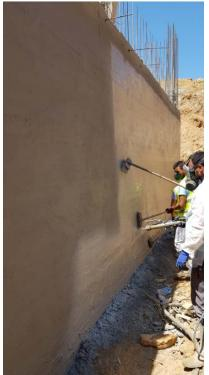
wimming pools, bathrooms & outdoors: Waterproofing of these surfaces was performed using the 1-component cementitious mortar Sikalastic®-1K with crack bridging properties.
