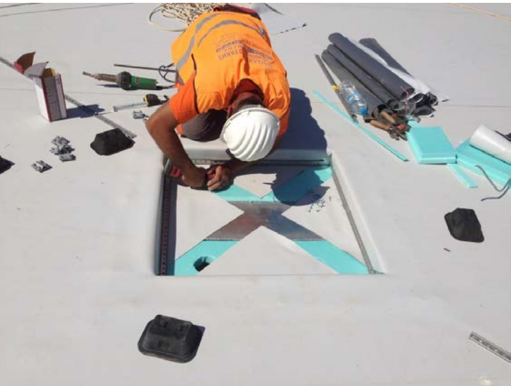
On the exit area towards the canopy, the adhered membrane Sarnafil® G410-12 EL was applied.
