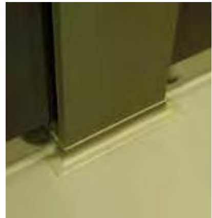
Floor-Wall Connection with Sikafloor® and SikaGard® WallCoat.
