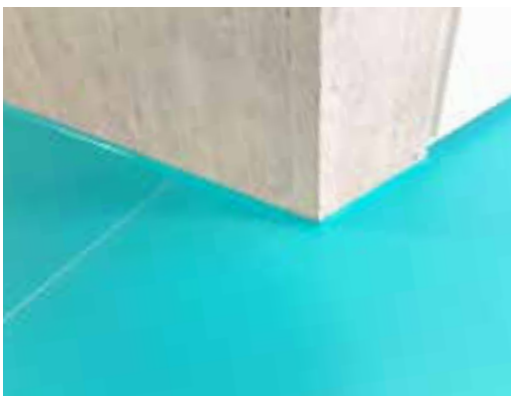
Sikafloor® Joint Solution with Sikaflex® PRO-3.
