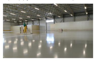
Joint sealing was performed using **Sikaflex® Pro-3**, a 1-component elastic polyurethane sealant featuring high mechanical and chemical resistance. In addition to its high movement capability, it features special particulate emission & biological resistance certificates and special certificate for suitability for use in food processing facilities.
