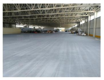
Special notch joints were then formed to anchor the system perimetrically and around details (e.g. pipettes) and then a scratch coat was applied using **Sikafloor®-210 PurCem**. The application was completed by laying the **Sikafloor®-210 PurCem** base layer.
