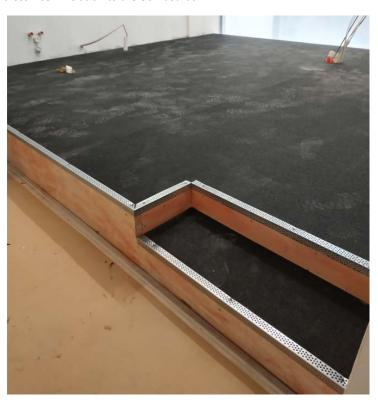
**Sikafloor® Comfort® Adhesive** (adhesive layer) was applied on this formed substrate, on which the **Sikafloor® Comfort® Regupol 6015 H** antishock pad was laid. This was followed by the application of the self-leveling, polyurethane-based resin **Sikafloor®-330**. The system was completed with the application of colored, matt polyurethane-based surface protection layer and low volatile emissions, **Sikafloor®-305 W**.
