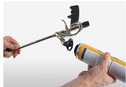
3 Screw Sika® RoofBond can into Spray Application Gun
