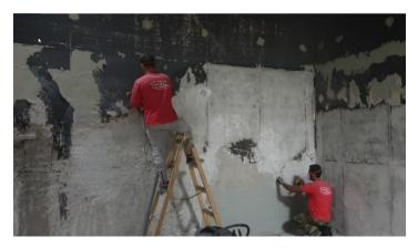
Application of **Sikagard®-720 EpoCem®** was followed by application of **Sikalastic® Primer MP** epoxy primer. **Sikalastic® Primer MP** offers excellent adhesion to prepared concrete surfaces, as it forms a gap and hole free surface. It has 100% solid content, without volatile organic compounds.
