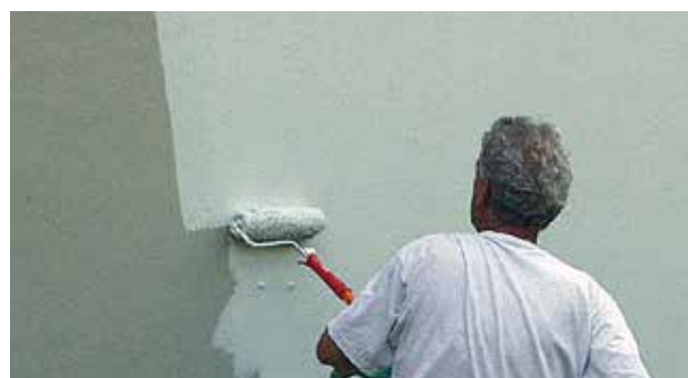
Epoxy resin-based protective coatings are applied over the entire surface following reprofiling of the concrete surface with sulfate-resistant repair mortar enhanced with synthetic material.
