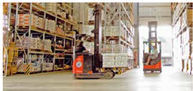
Industrial flooring surfaces also experience strong abrasion due to constantly rolling and striking loads in the same places. Hard concrete coatings and special dispersants can enhance the flooring grip and minimize wear.
