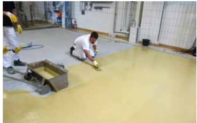
SATURDAY AFTERNOON: Application of the Sikafloor® PurCem® HM-20 hybrid polyurethane flooring.
