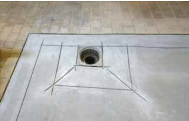
SATURDAY MORNING: Substrate preparation after curing of the screed.
