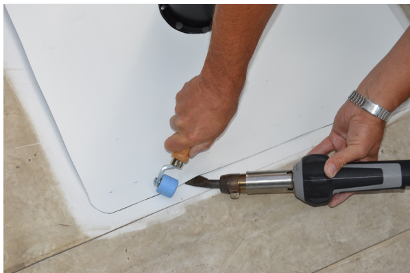
7. Application of pipe flashing
