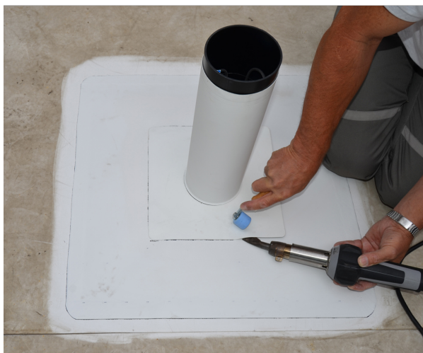
8. Finished installation of Sarnafil® T RCS Set complete
