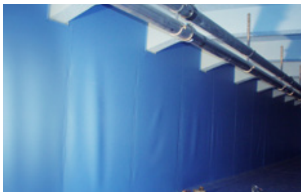
WATER RESERVOIR ZOLLERNALB, GERMANY 2006
