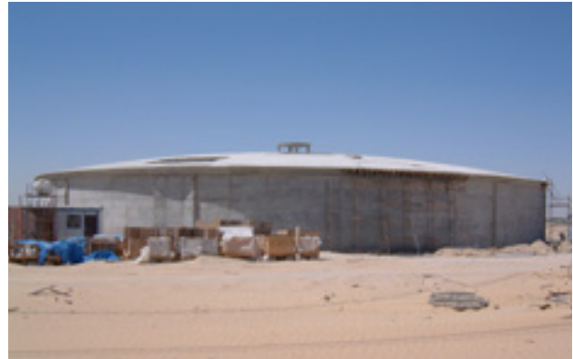
AL AJBAN WATER RESERVOIR, ABU DHABI, U.A.E. 2003
