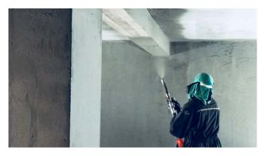
**Sikagard®-720 EpoCem®** carries a Declaration of Performance as Concrete protection product – Coating (EN 1504-2) and as PCC Class R4 repair mortar (EN 1504-3).
