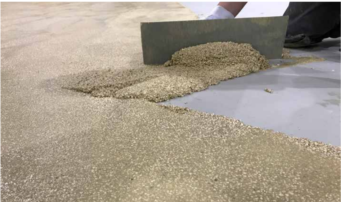
Sikafloor® PurCem® HM-20 HSR is a textured trowel-grade system with high slip resistance. Typical application is done with a trowel or “screed box.”
