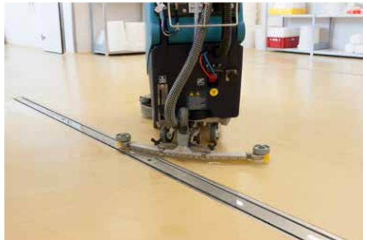
Sikafloor® PurCem® HM-20 in an ice cream plant.
