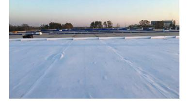
The special automatic welding machine **Sarnamatic®** was used to weld the membrane.
