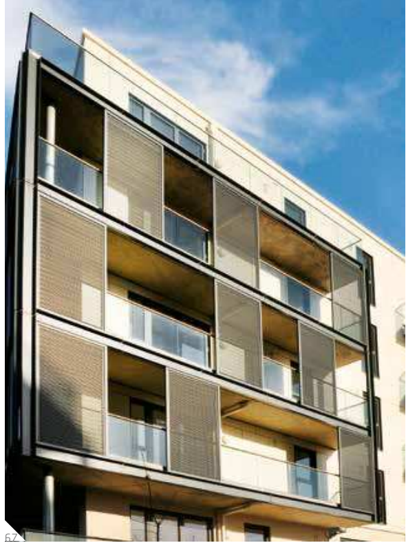
67 67 Threshold Residential, Parsons Green, London Client: Threshold Housing Association (UK) Facade by Cladding UK
