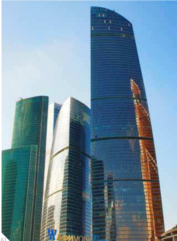
61 Russia Federation Towers, Moscow (2008) Architects: Tschoban & Schwegler (DE) Facade by Shenyang YuanDa (CN) Insulating Glass by SYP (CN)
