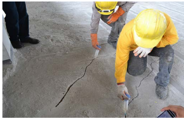
Non-moving crack repair. Opened crack is filled and injected by using Sikadur®-52 or Sikafloor®-156 epoxy resin.
