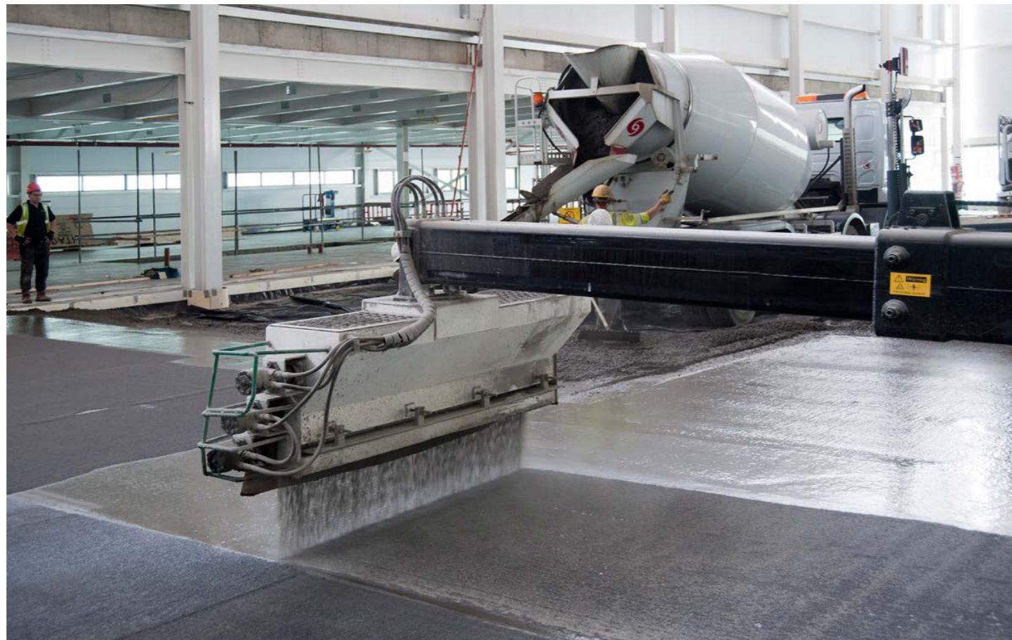
Mechanical spreading of Sikafloor®-2 SynTop dry shake hardener on fresh concrete.
