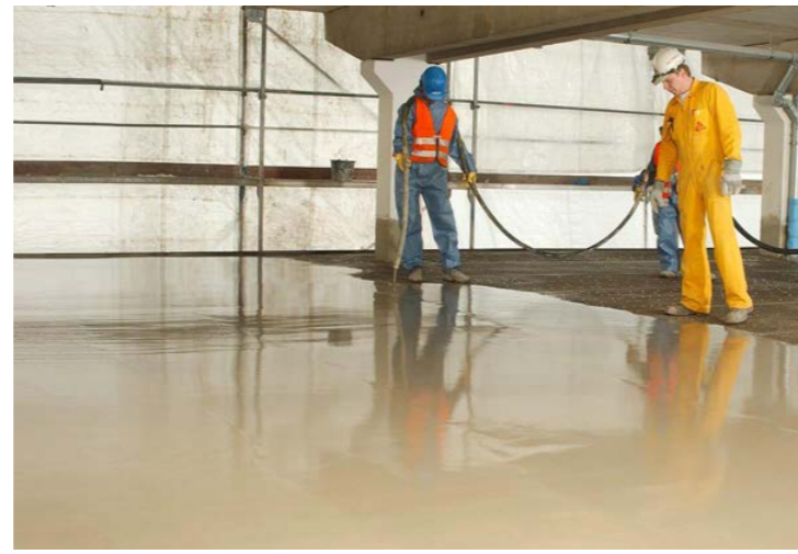
Application of Sikafloor®-30 Level overlay in a parking deck.
