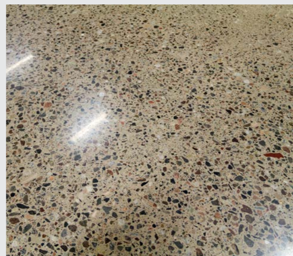
Aggregate finish grinding with Class 4 polish level. Source: HTC Professional Floor Systems.
