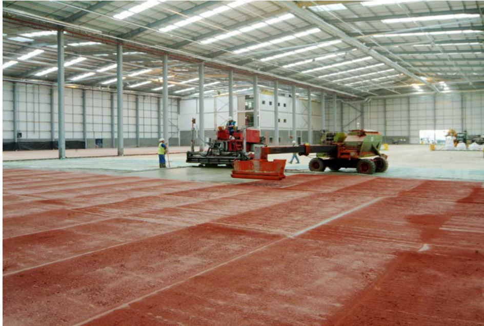
Colored Sikafloor®-3 QuartzTop application.
