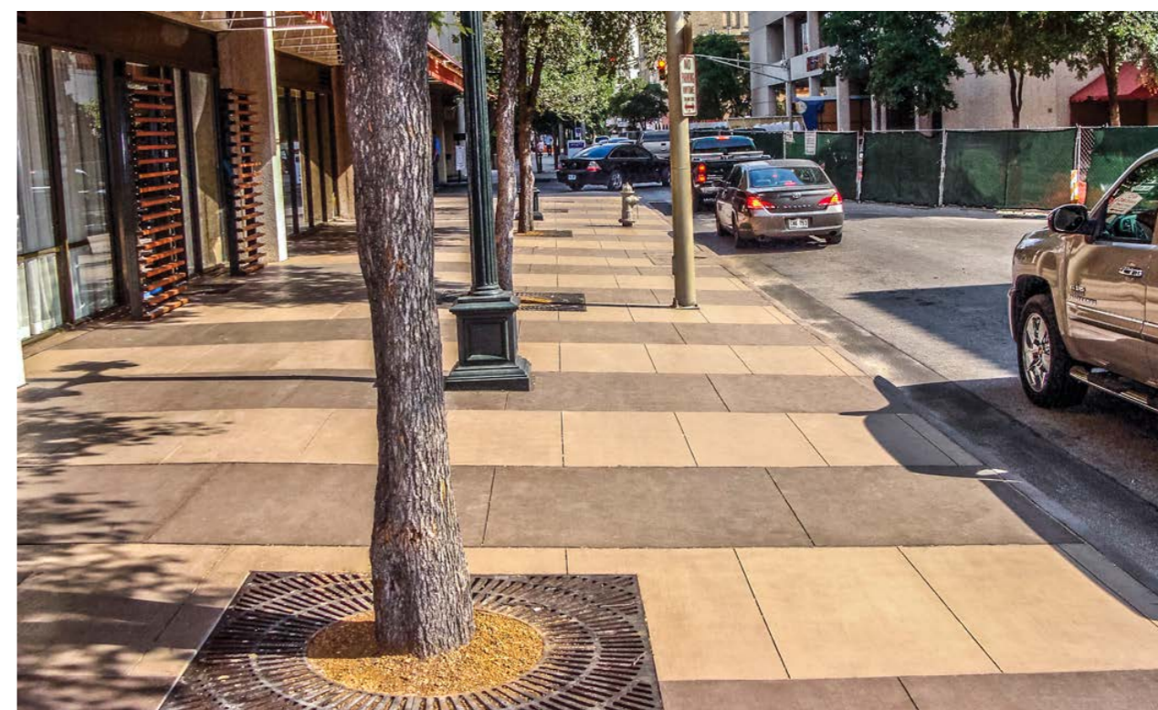
Integral colored pavement with Sika® concrete colorant.
