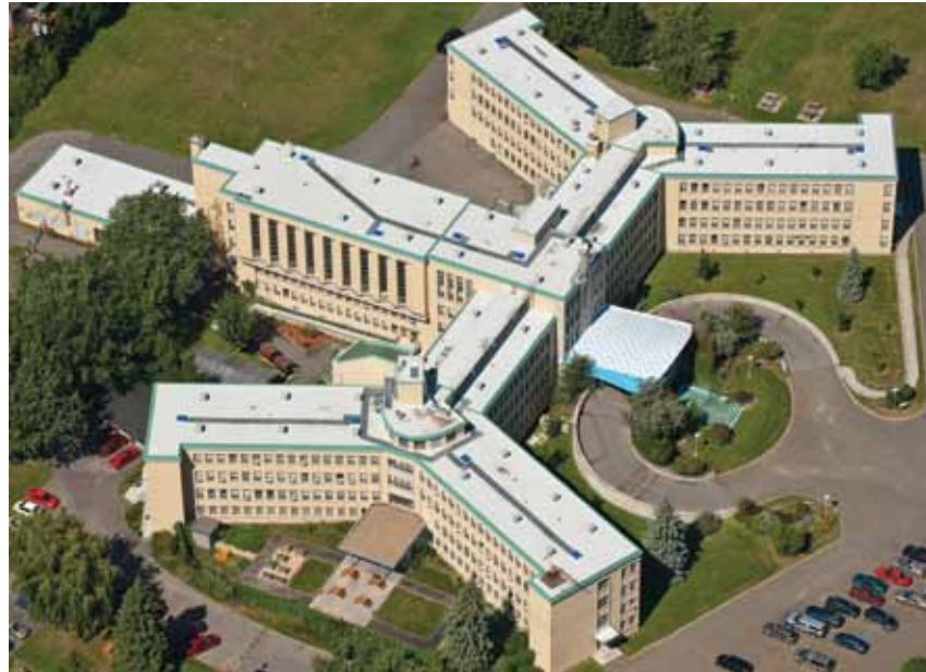
▲ Le Foyer Rousselot, a long term care facility in Montreal, Quebec that is affiliated with the Lucille-Teasdale Health Centre, chose to cover its unique roof with a combination of G410-15 and G410-20 Sarnafil® EnergySmart Roof membranes.
