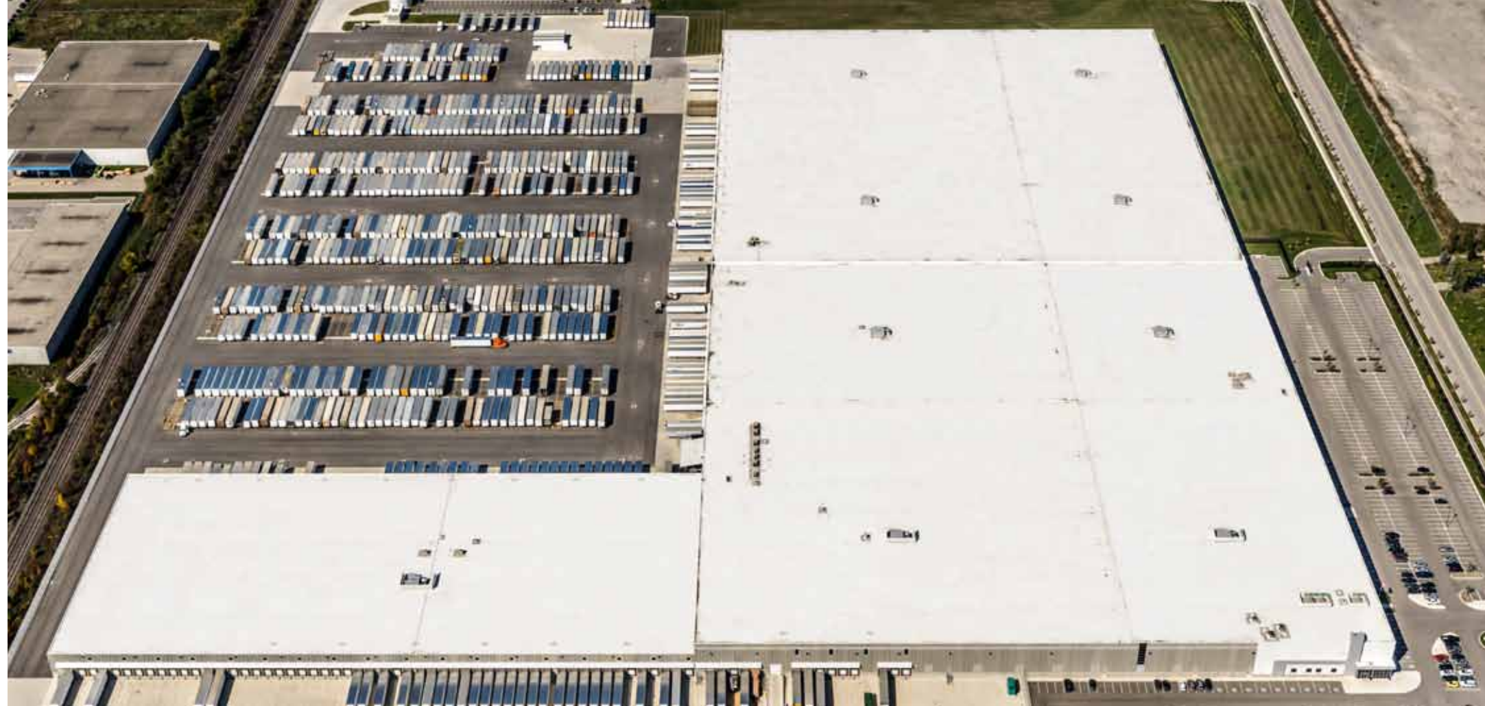
▲ A reflective Sika roofing membrane was selected to cover the 1.3 million square foot Target Distribution Centre in Milton, Ontario
