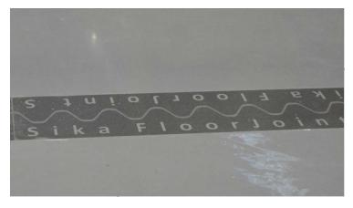
The profiles are placed at the same level as the floor, which means that there are no steps and uneven spots. A further advantage of this new system is the minimized damage to vehicles, which entails significantly reduced spare parts. It is really a value-added solution in every respect.
