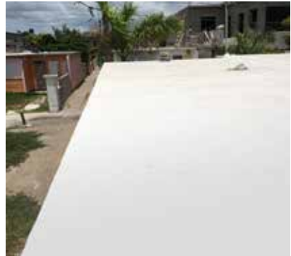
Fig. 5. Finished roof with 3 coats of Sikalastic®-560.
