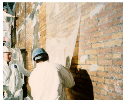
SEISMIC UPGRADING /EARTHQUAKE DAMAGE REPAIR
