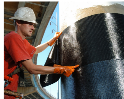
SikaWrap® fabrics also including: Aramid Fibre Fabrics, Special Bidirectional and Quadraxial Fabrics
