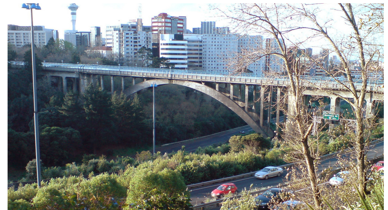
Grafton Bridge, Auckland, New Zealand
