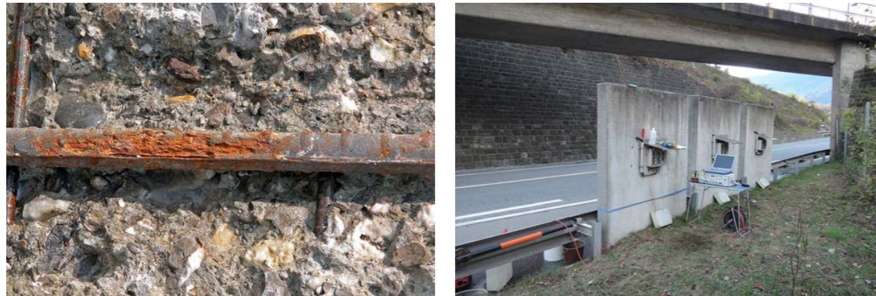
Damage to concrete structure due to insufficient concrete cover and low concrete quality.
