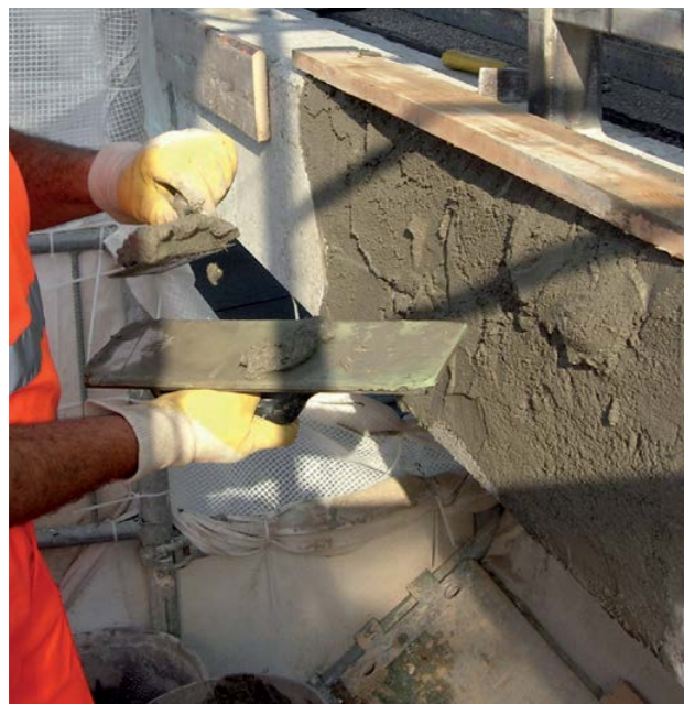
Hand applied mortar
