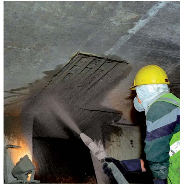
Sprayed mortar
