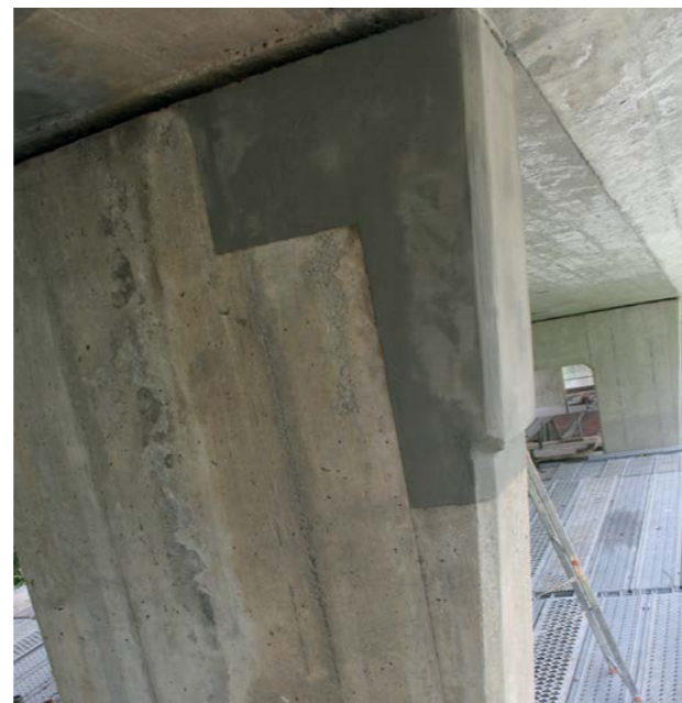
Repair work completed
