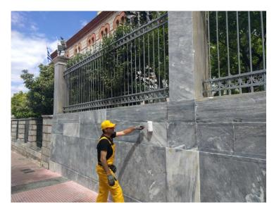
The primer layer was allowed to dry and become touch-dry (tack-free) prior to the application of second coat (~3 hours between the layers) The second and final coat of **Sikagard®-850 AG**, diluted with a small percentage of white spirit, was also applied using roller and brush.
