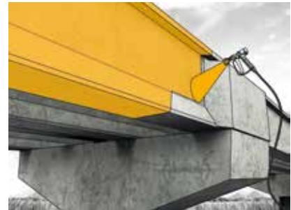
Machine applied using airless spray.
