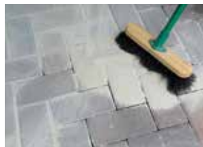
2. Brush into the joints
