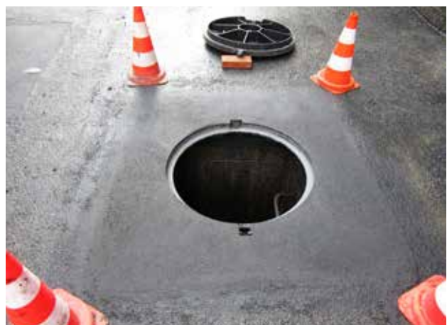
Finishing of Sika® FastFix-138 TT before it hardens.
