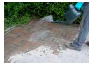
4. Saturate the surface and the joints with water using a hose or watering can.
