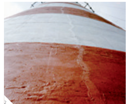
1 Structural bonding of cracks to restore structural integrity with Sika® Injection resin. 2 Crack-sealed with Sikaflex sealant and overcoated with Sikagard®-680 S protective coating.
