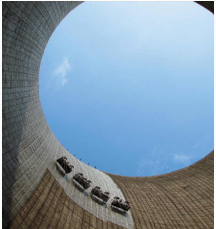
Application of the Sika Icosit®-2406 protective coating system from specialist powered access cradles.
