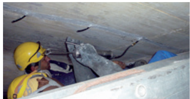
Crack Injection.
