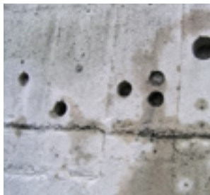
Quality control of the concrete. Core drilling on the wall.
