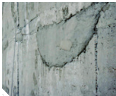
1 Hand applied Sika MonoTop® repair mortar.
