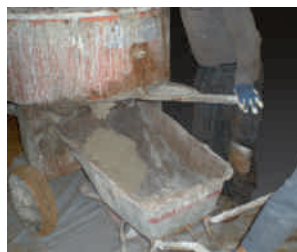
Mixing of Sikafloor® Marine KG-202 N and KG-404 N
