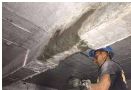
Concrete repair and refurbishment, Page 28
